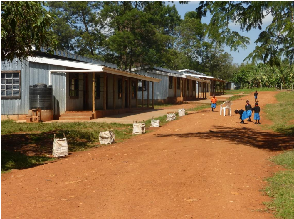
Open Arms Academy Classroom Blocks
